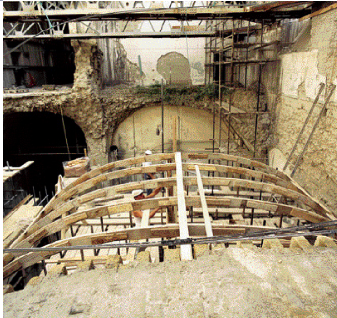
A CORRIDOR ON THE TOP FLOOR, TOP, HAS A NEW TIMBER ROOF. PARTS OF THE BUILDING, ABOVE, HAVE BEEN BRACED TO PREVENT COLLAPSE. RIGHT, VAULTS ARE UNDER CONSTRUCTION, FOLLOWING THE TIMELESS TECHNIQUES OF TIMBER VAULTING AND USE OF LOCAL VOLCANIC TUFA STONE.
