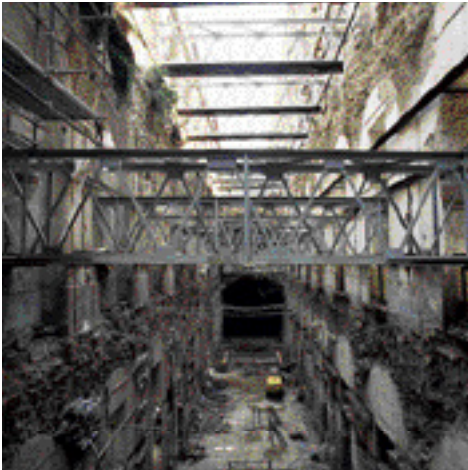
A CORRIDOR ON THE TOP FLOOR, TOP, HAS A NEW TIMBER ROOF. PARTS OF THE BUILDING, ABOVE, HAVE BEEN BRACED TO PREVENT COLLAPSE. RIGHT, VAULTS ARE UNDER CONSTRUCTION, FOLLOWING THE TIMELESS TECHNIQUES OF TIMBER VAULTING AND USE OF LOCAL VOLCANIC TUFA STONE.
