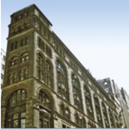
CORBIN BUILDING, NEW YORK
