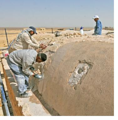
Conservation of the exterior of the site. Application of a lime mortar layer
