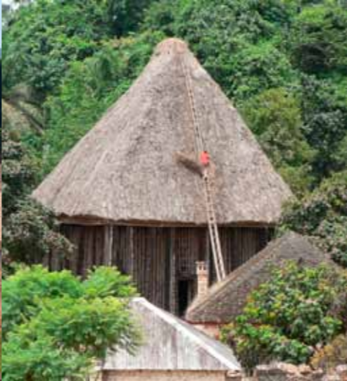
Restoration work on the roof of Achum shrine
