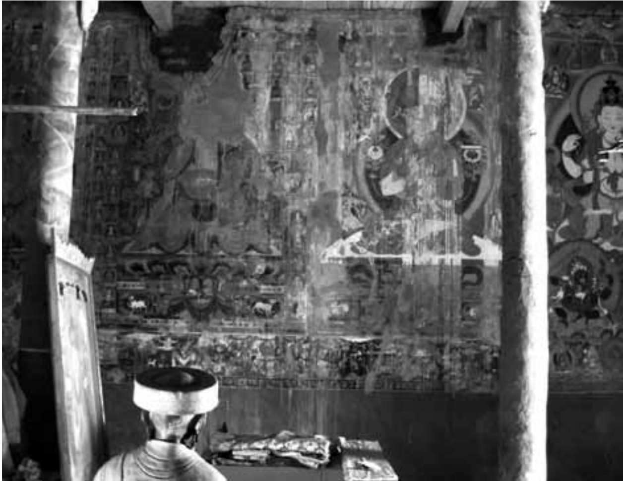
Badly damaged temple murals depicting the Buddhist pantheon had to be restored to reinstate the spiritual sanctity of the images
