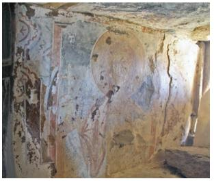
FIGURE 132 Deterioration around window opening on the south wall of the church
