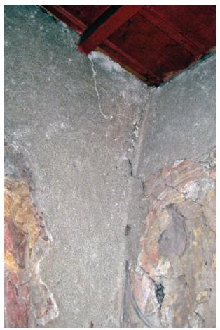
**FIGURE 31** Interior wall damage resulting from previous deterioration and subsequent repairs
