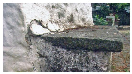
Mock-up bench prior to the implementation of work. Note the ungainly cement cant at the rear of the seat, and biological growth.
