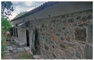
**FIGURE 119** Leaves in the sunken walkway contribute to water retention near the church
