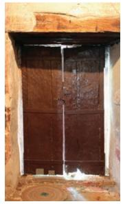
FIGURE 37 Door D1, from the interior, showing steel batten straps
