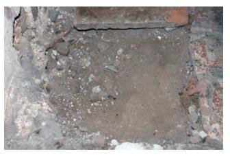
FIGURE 67 Floor tiles and soil substrate in the narthex
