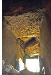
FIGURE 56 Stone lintel above the recessed window opening, view from the interior
