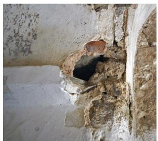
FIGURE 107 Void in the masonry
