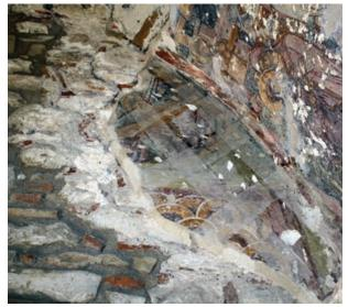
FIGURE 109 Wall paintings stabilized using fabric
