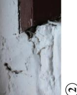
Surface cracking is also common at the interface between lintels or tends to be superficial cracks in stone and mortar wall. There headers and the surrounding the mortar or whitewash.
