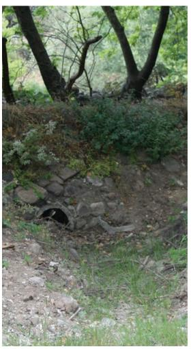
FIGURE 12 The drainage channel flows through a pipe into the Voulgaris River.
