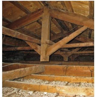
FIGURE 33 Main roof wood framing
