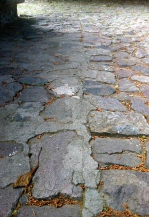
FIGURE 16 Open joints between the stone pavers filled in with hydraulic cement
