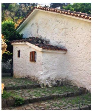
FIGURE 28 Although the interior floor level remains constant, the raising of the exterior grade at the east façade is very damaging
