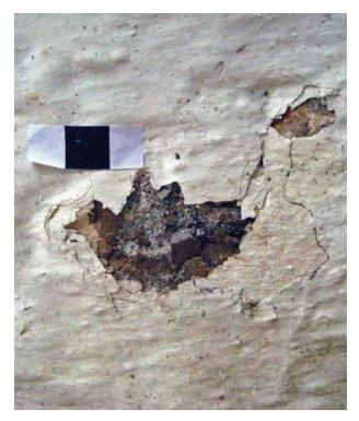
FIGURE 27 Small *lacunae* in the exterior lime finish are easily repaired. Exterior finishes are in good condition
