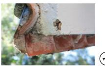
Rebar placed close to the surface has causing spalling. oxidized and is
