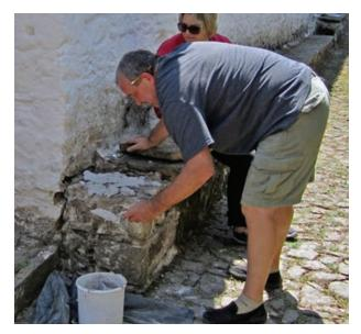
5. The mortar was hand-troweled onto the top of the bench.
