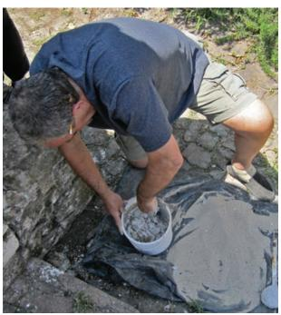
4. The new mortar was mixed at an approximate 1:3 limeto-sand ratio, and water was added to achieve the proper consistency.
