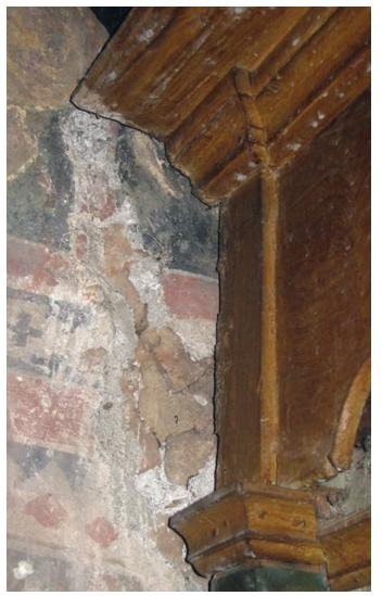
**FIGURE 76** Evidence of deterioration at the cornice of the iconostasis
