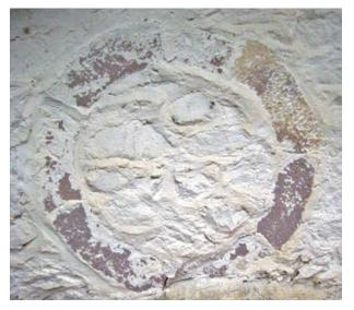
FIGURE 23 The rose window on the east façade has been filled in
