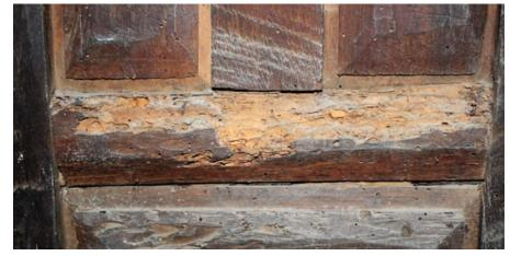
FIGURE 48 Evidence of insect infestation on the unpainted side of the door
