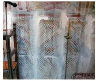
FIGURE 124 Evidence of damage from seating furniture
