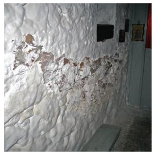
$\ensuremath{\textbf{Figure 101}}$  Spalling plaster on the north wall of the church
