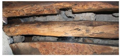
FIGURE 52 Detail of lintel showing insect flight holes
