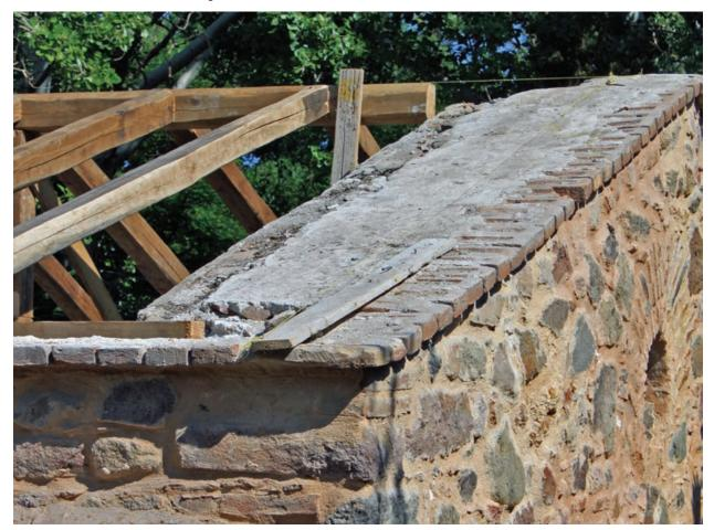
FIGURE 127 Soffit capping the top of the walls of the church
