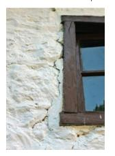
FIGURE 59 Detail of loose lime-based mortar around window trim, view from the exterior
