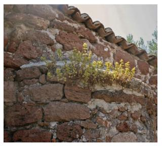
FIGURE 99 Plant growing on the north apse of the triconch
