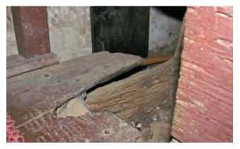
FIGURE 69 The concrete floor slab does not extend underneath the Bishop's throne
