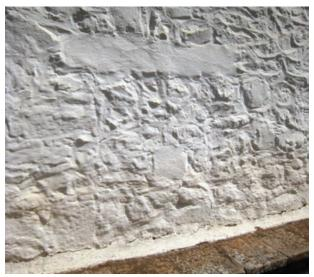
FIGURE 24 A former door opening on the south façade has been filled in
