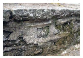
**FIGURE 30** Hard hydraulic cement mortar at benches entraps water, exacerbating wall deterioration
