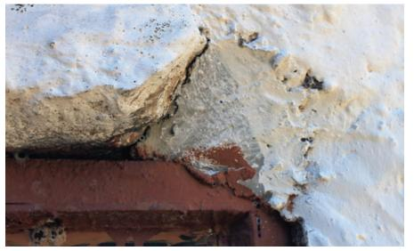
FIGURE 55 Hydraulic cement patching on the top right corner of the stone lintel
