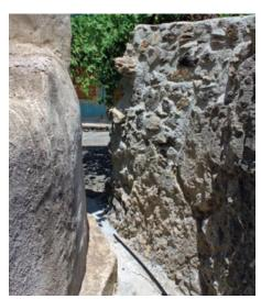
FIGURE 113 Separation trench between the east side of the church and the adjacent hillside
