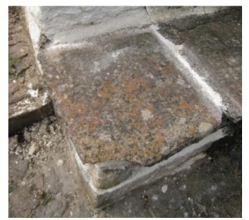
Completed repointing with reduced cant, new limewash on adjacent wall, and new mortar joints
