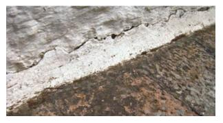
FIGURE 25 A hydraulic cement cant at the bench edges entraps moisture. Note the typical gap at the rear upper edge, a result of differential expansion and contraction.
