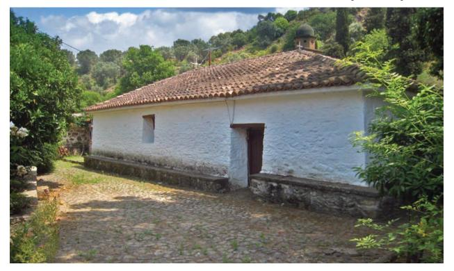
FIGURE 19 The building is rectangular in plan, with the longer side running east to west Investigative probes revealed that the walls extend at least 40 centimeters (16 inches) below grade, and appear to rest directly upon the soil substrate (Figure 20). Probes were performed on interior faces of the west exterior wall within the narthex, and within the Sanctuary, at the wall separating the Sanctuary and the narthex.
