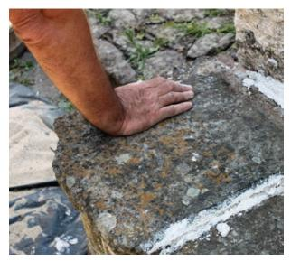
7. The bench seat was set in the new mortar so that the seat sloped slightly to the front of the seat, to achieve proper drainage. A new smaller cant was applied to the rear edge of the seat.
