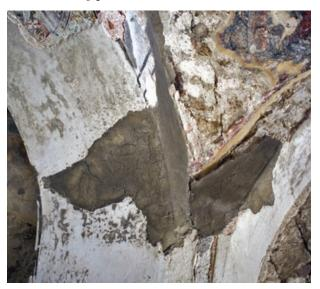
FIGURE 108 Inappropriate repairs using cement
