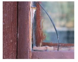
FIGURE 65 Exterior sash detail, showing missing glazing compound and cracked glass
