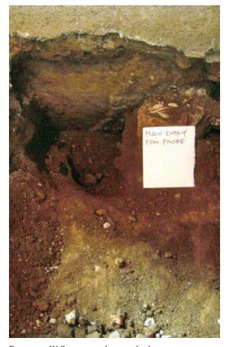
FIGURE 20 Walls penetrate the ground at least 40 centimeters, but lack footings
