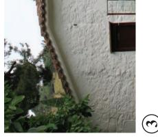
wall that separates the nave and There is significant separation narthex indicating the narthex corresponding to the interior is an addition.
