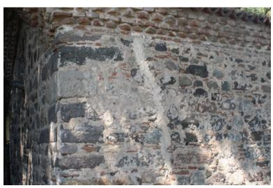
FIGURE 135 A large crack runs through the south wall
