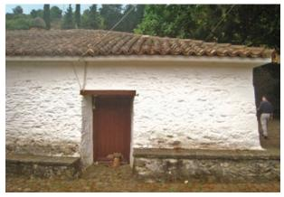
FIGURE 22 "Battering" of the stone masonry walls suggests dry-laid stone construction
