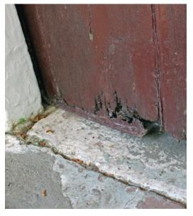
FIGURE 38 Wood deterioration from moisture at the bottom of Door D1
