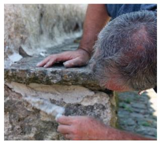
8. The mortar joints were repointed in two lifts, and after a short amount of time were tooled to match the adjacent joint tooling, with a slight "ridge" at the center of the joint.
