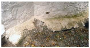
FIGURE 26 Walls lacking exterior benches meet the ground with a hydraulic cement cant
