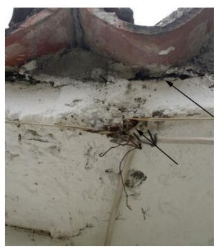
FIGURE 35 Cracking and deterioration due to rusting rebar
