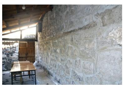
FIGURE 137 The north wall has been covered with cement mortar
