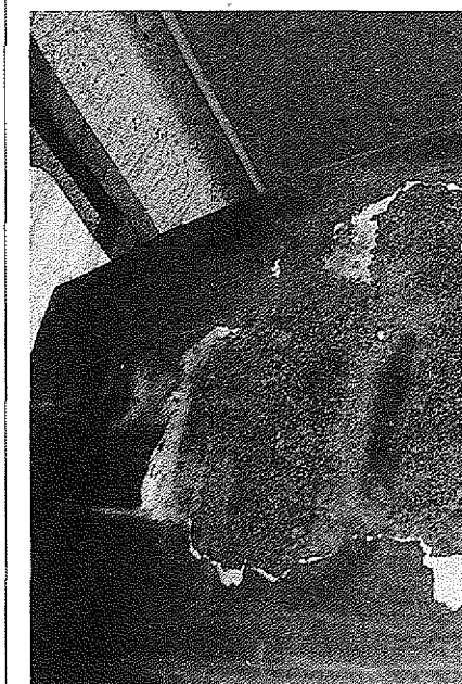
DETAIL SHOWING CORROSION ON ONE MODULE OF BRANCUSI'S ENDLESS COLUMN , PRIOR TO CONSERVATION TREATMENT AND REASSEMBLY.
