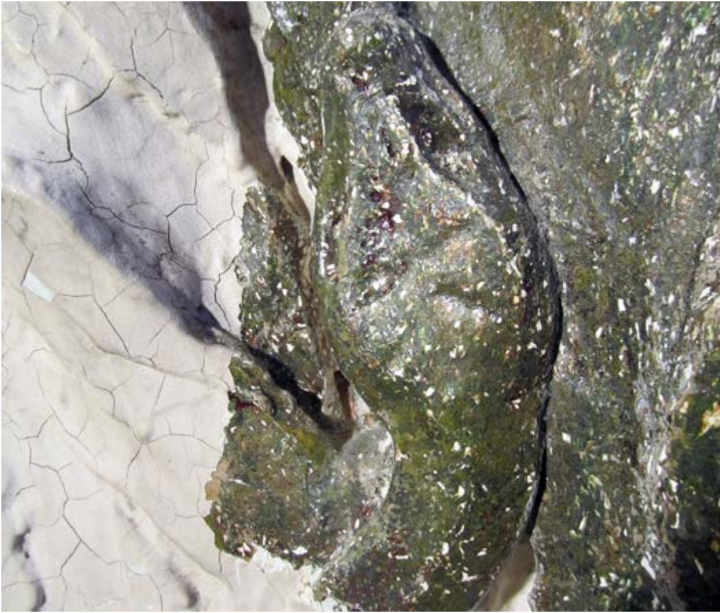
Layers of white paint were removed from a section of the fireplace, revealing Chanler's original finishes
