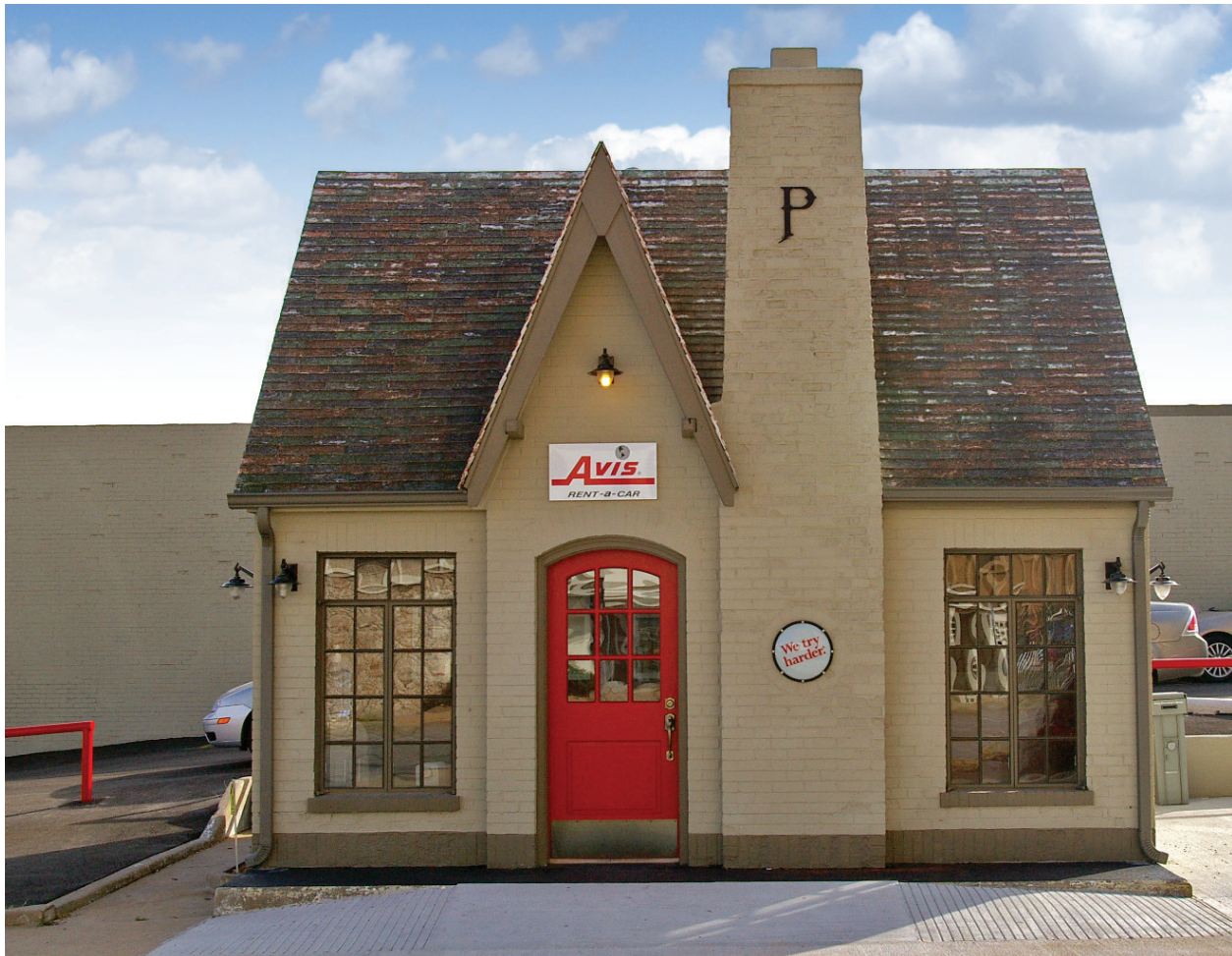
Built in 1932, Vickery Station is an intact example of the “Cotswold Cottage” design used by Phillips Petroleum Company
