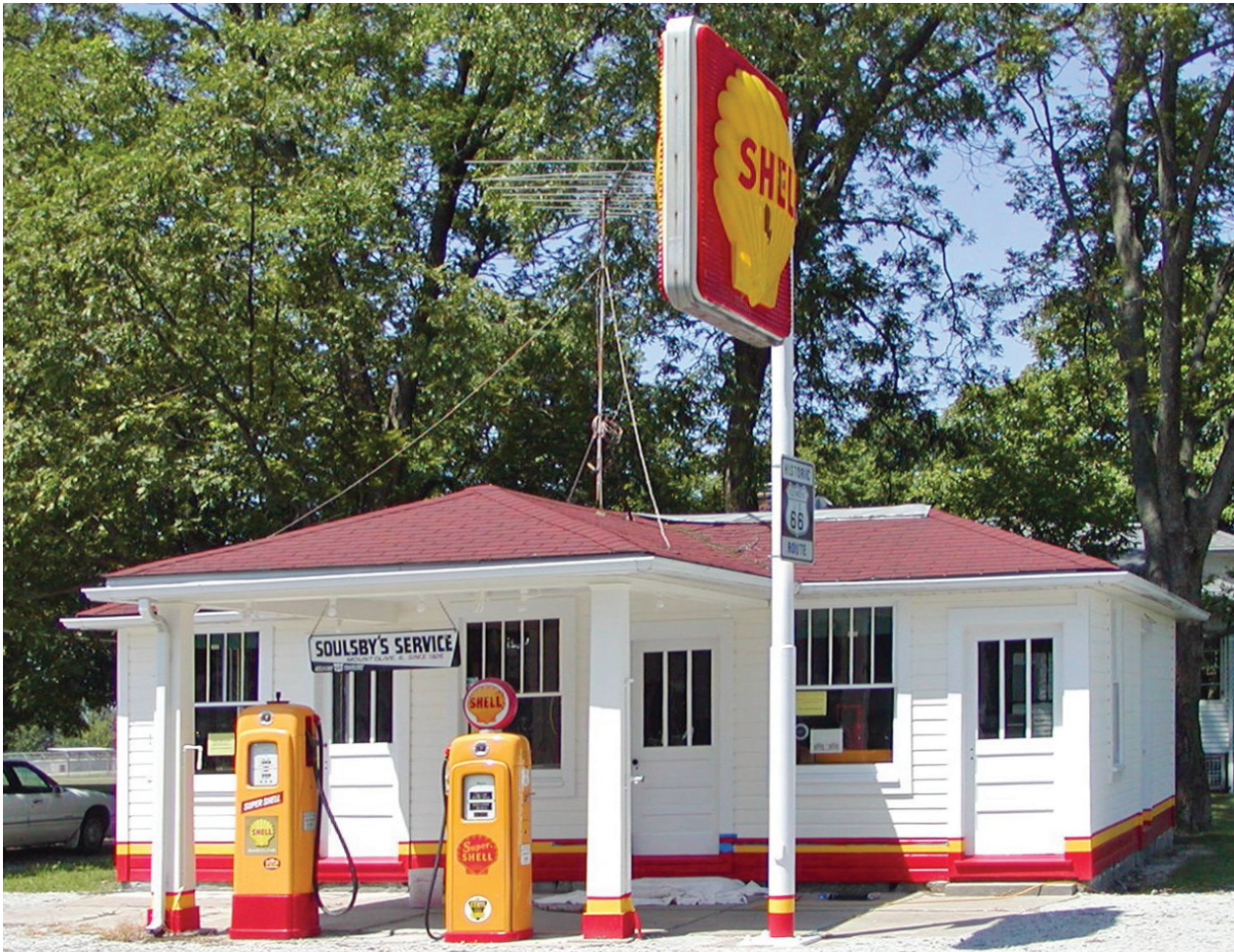
Built in 1926 by Henry Soulsby, this Shell station is one of the oldest still standing on Route 66
