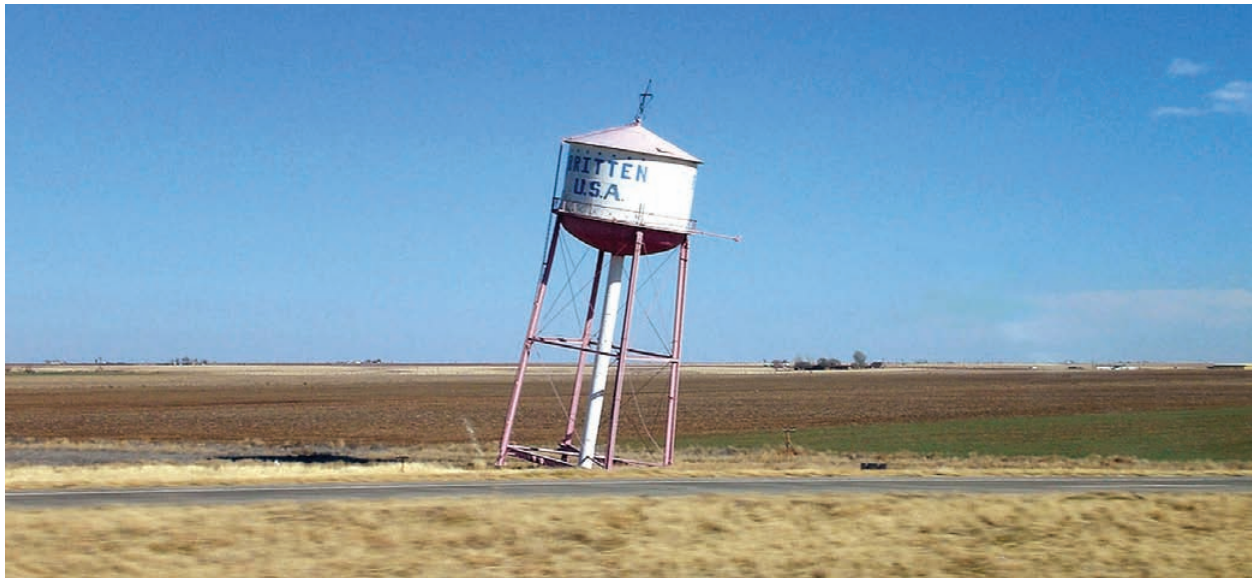
The Leaning Water Tower along Route 66 near Groom, Texas
