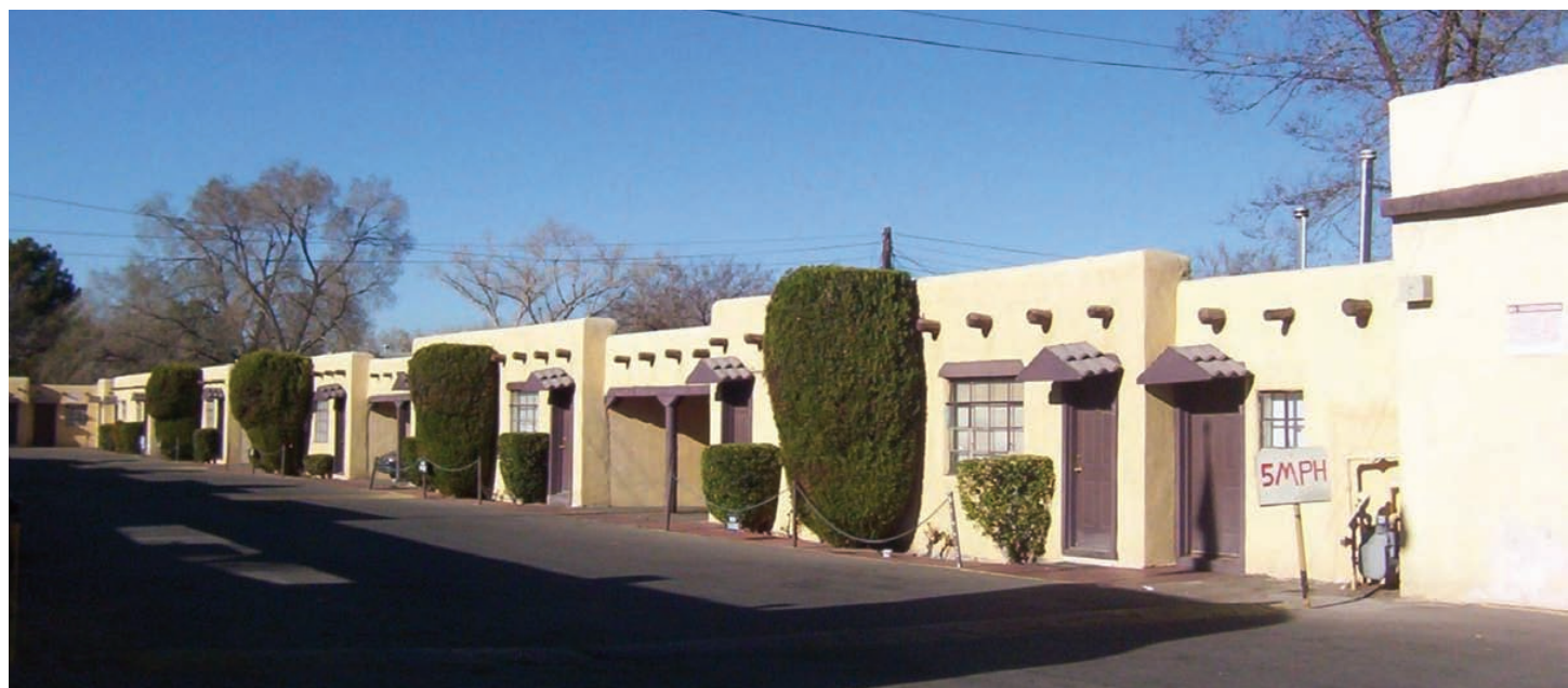
Horn Lodge in Albuquerque, New Mexico, was demolished for condominium development in 2006
