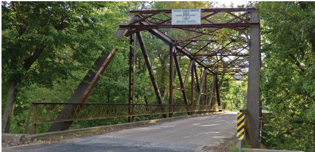
The Pryor Creek bridge, just east of Chelsea, Oklahoma
