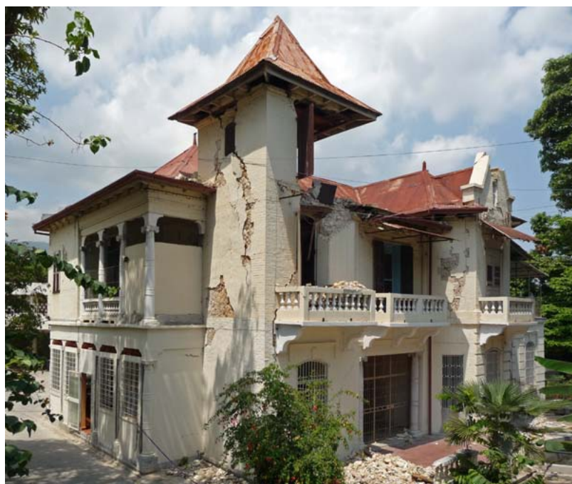
FIGURE 3 The Catholic seminary at 110 Rue Fleur Du Cheine. This masonry bearing-wall structure exhibits partial collapse of corner tower.
