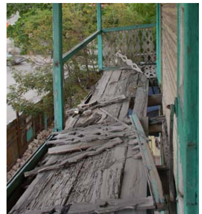
FIGURE 78 Second-floor porch structure made unsafe by termite damage.
