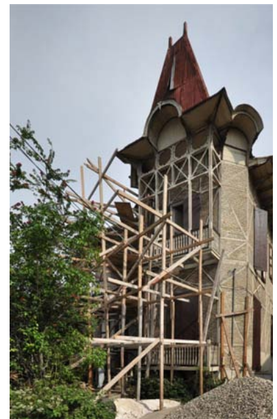
FIGURE 120 Scaffolding and shoring at 32 Lamartiniere, and shoring on the interior of 22 Rue Pacot.
