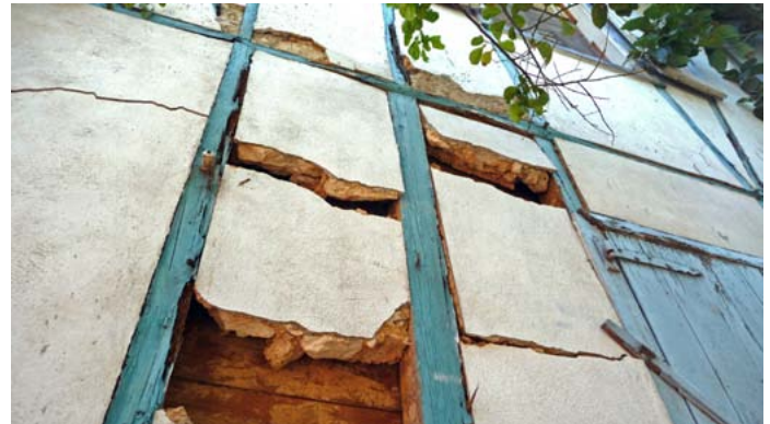
FIGURE 39 Colombage at 5 Rue Jose Marti with limestone and earth mortar infill, with lime plaster finish. Interior board sheathing can be seen.
