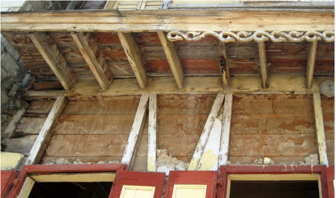
FIGURE 66 Poor construction and detailing have made many balconies vulnerable to decay and structurally unsafe. For those balconies supported on the cantilever extension of the floor joists, decay can extend into the house, putting both the balcony and interior floor at risk.
