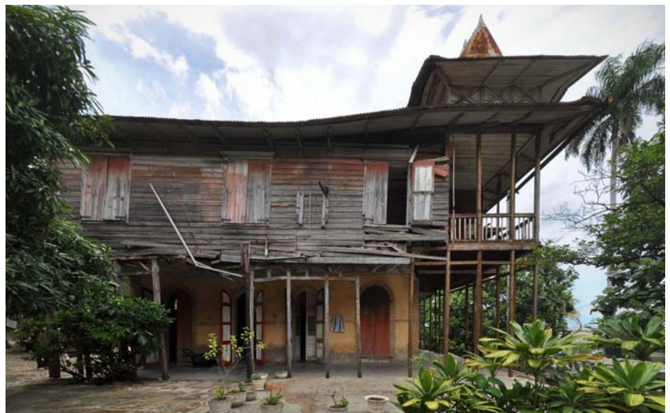
FIGURE 65: The Patrice Pamphile House (shown also in Figures 2 and 32) showing the heavily deteriorated wooden part of the structure, which at one time probably had been an open porch.
