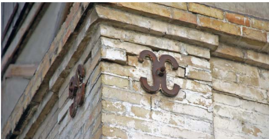
FIGURE 26 View of decorative end plates at the corner of this brick structure indicate horizontal ties along each wall of the intersect.
