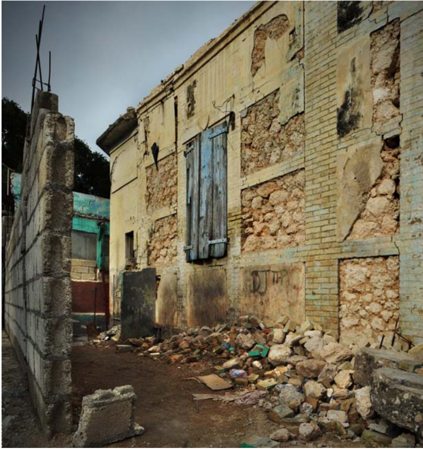
FIGURE 45 left Wall of a commercial building on Avenue Lamartiniere showing the characteristic layout of the mixed brick with rubble stone masonry found in many Gingerbread houses in Port-au-Prince. The brick piers and horizontal brick courses are crucial in restraining the walls from complete collapse. right Interior view of wall of the Villa Castel Fleuri (see Figure 1) showing a rubble stone panel which has completely collapsed out from between the brick masonry piers. Notice the brick keys that had extended into the rubble stone panel.
