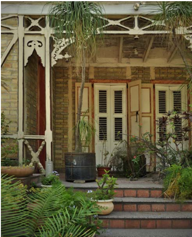
FIGURE 36 79 Avenue Christophe showing colombage with brick infilling.
