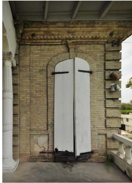
FIGURE 108 The Villa Castel Fleuri shows the effect of the absence of iron chains at the 2nd floor level corners. The pier on the right has been slightly displaced to the right at the second floor level. It is possible to repair it without rebuilding it, but the deflection will then remain visible. A better quality and more resilient restoration will require shoring and relaying of the masonry of the corners of the building with new masonry units to replace the rubble stone. The rebuilt masonry need only extend across to about the middle of the arch.
