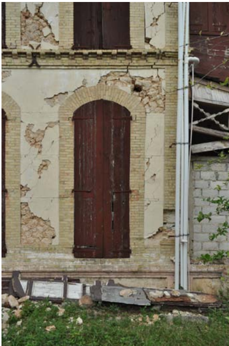
FIGURE 108 The Villa Castel Fleuri shows the effect of the absence of iron chains at the 2nd floor level corners. The pier on the right has been slightly displaced to the right at the second floor level. It is possible to repair it without rebuilding it, but the deflection will then remain visible. A better quality and more resilient restoration will require shoring and relaying of the masonry of the corners of the building with new masonry units to replace the rubble stone. The rebuilt masonry need only extend across to about the middle of the arch.
