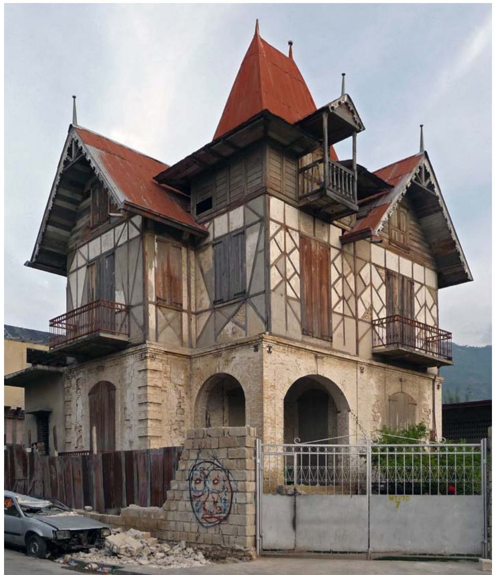
FIGURE 49 Hybrids are very common. This Gingerbread house at 59 Lavaud 3 utilizes all three wall-construction systems: Attic walls—wood frame Second story—colombage First story—masonry bearing wall Note also the one-story concrete addition at the back left corner.
