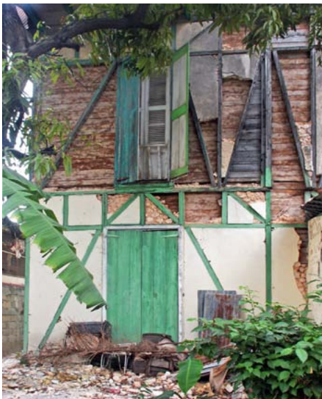
FIGURE 86 Much of the colombage stonework fell out of the walls of the second story during the earthquake.
