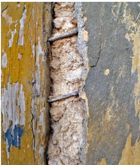
FIGURE 43 Nails help hold the earthen infill.
