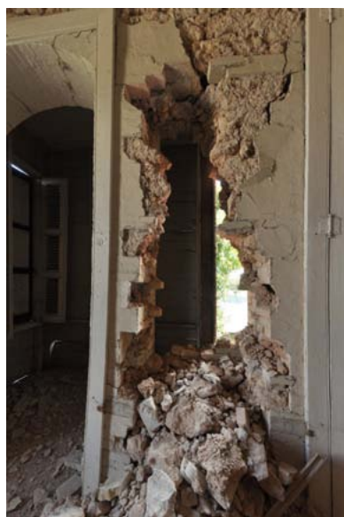
FIGURE 130 below left A rubble panel on the second floor of the Villa Castel Fleuri that collapsed showing the displacement of the bottom of the brick pier into the doorway which resulted from the expansion forces from the panel. below right Le Manoir on Avenue John Brown showing a heavy level of disruption of the masonry walls caused by the rapid degradation of the rubble stone panels during the earthquake.
