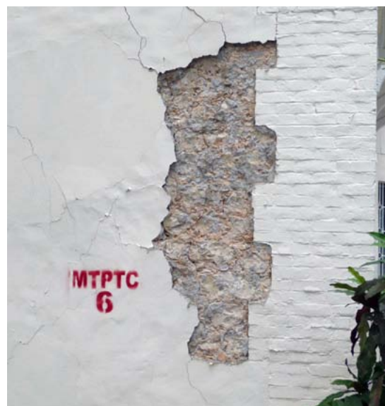
FIGURE 4 The red painted designation “MTPTC 6” indicates that inspection deemed the tower unsafe for occupancy by the Ministère du Travail Public et Télé Communications.
