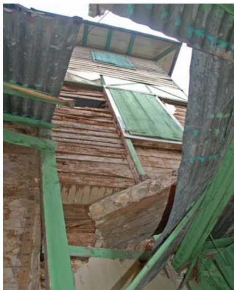
FIGURE 89 Brick infill that had been relaid with cement mortar fell out in huge pieces during the earthquake, causing damage to construction below.
