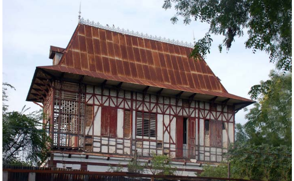
FIGURE 55 Corrugated ferrous metal roofs are quite common on the Gingerbread houses. This house has a metal crest at the ridge as well.
