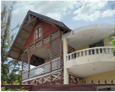
FIGURE 48 Concrete additions are often awkward or compromise the Gingerbread buildings architecturally, like this one at 51 Avenue Christophe.
