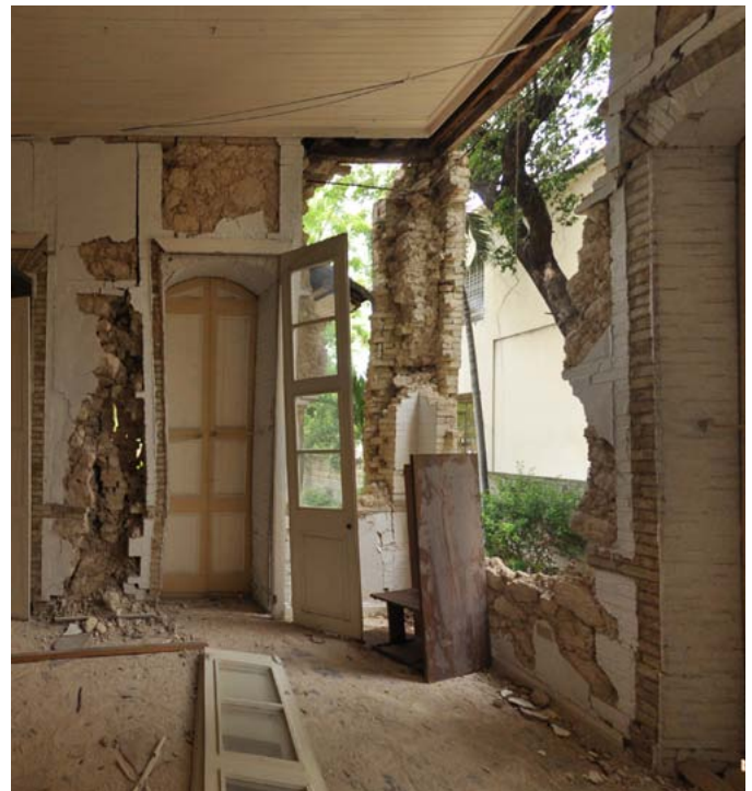
FIGURE 95 above left The Dufort House showing the collapse of the rubble panels, leaving the piers standing holding up the almost undamaged upper floor structure. The remarkably large pile in front shows the volume of rubble masonry removed from the house after it had collapsed. above right The interior of the Dufort House, also shown in Figure 77, showing how the collapse of the rubble panels left the house standing on the brick piers which were left like free standing columns. left This house also had steel or wrought iron reinforcing chains made up of rods hooked together for the full length of the exterior and major interior walls. In this case, rather than exterior plates to hold them, their wall anchors were imbedded under the outer wythe of masonry. The rods are also visible where they intersect at the corner pier that is still standing, which can be most clearly seen in Figure 93.
