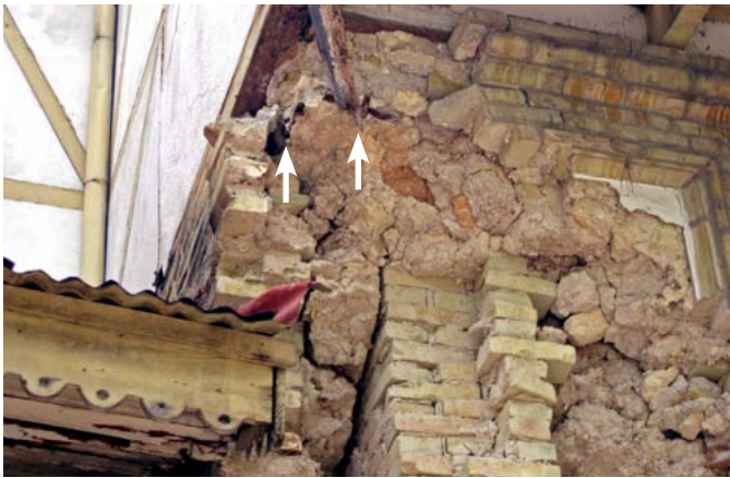
FIGURE 103 Embedded tie rods cross at the corner, anchored by iron bars. Also note rubble fill between inner and outer leaves of brick masonry.
