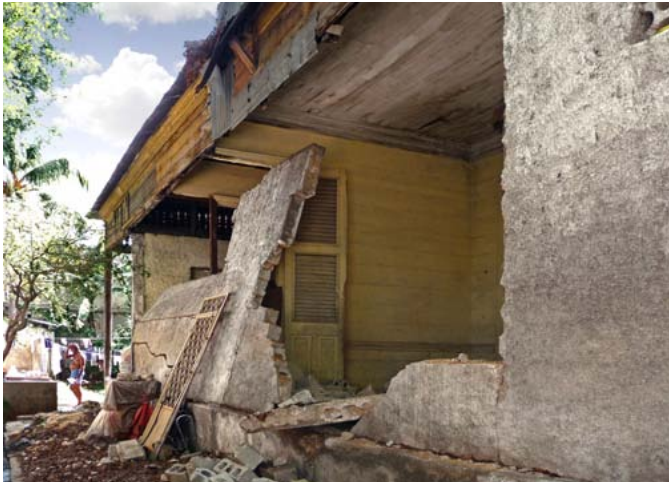
FIGURE 72 A replacement side wall of concrete block at 19 Lamar-tiniere suffered partial collapse.
