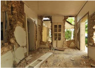
FIGURE 94 Ground floor interior of the Albert Dufort House on Rue du Travail Deuxième showing complete disruption of the rubble panels in its construction. The interior wall on the left, which did not have brick piers walls because of the lack of window and door openings, collapsed completely.
