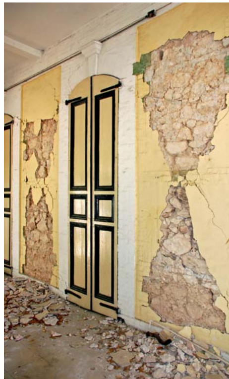
FIGURE 115 The characteristic X-cracks seen on masonry wall infills of concrete frames are also present at Le Manoir. These are due to the reinforced concrete second floor slab (above the damaged wall in this picture).
