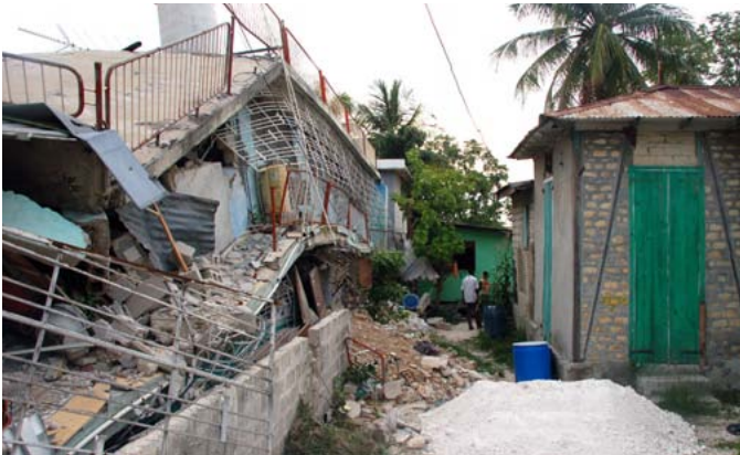
FIGURE 75 A pancaked concrete-frame building on the left and a colombage house on the right showing the comparative performance of these building types in a seismic event.
