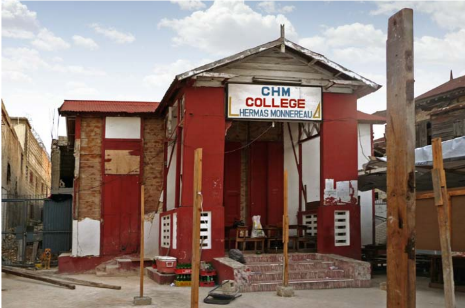
FIGURE 112 A small colombage school building at 16 Lamartiniere that had a two-story addition behind it. Large portions of this addition collapsed completely, but the original building is still intact and in use.
