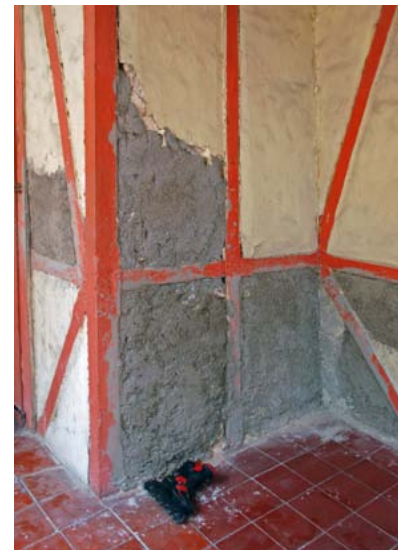
FIGURE 74 Improper repair of stone infill of colomage using concrete. These repairs constitute a fill that is much stiffer and more cohesive than the fill it replaced.
