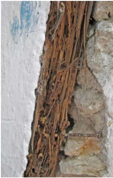
FIGURE 62 Termites thrive in Port-au-Prince, and many of the wooden structures are severely damaged due to termite attack.
