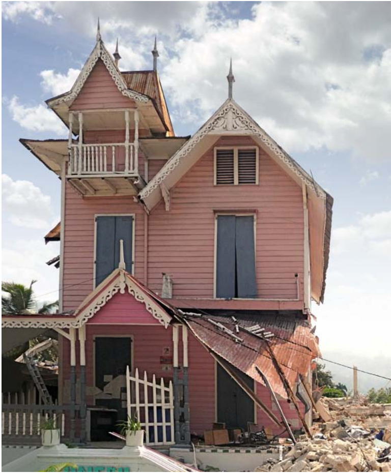
FIGURE 82 Wood frame Gingerbread at the Episcopal University at 14 Rue Légitime next to the site of a collapsed concrete building.
