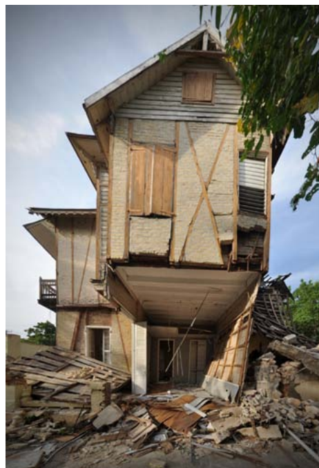
FIGURE 136 left House on Rue Jose Marti where the concrete addition collapsed, leaving the Gingerbread house cantilevered over the rubble. right The son of the owner of this house is pointing to the place where his cousin remains buried in the rubble of the collapsed concrete addition. This house is also shown in Figure 111 on page 52.
