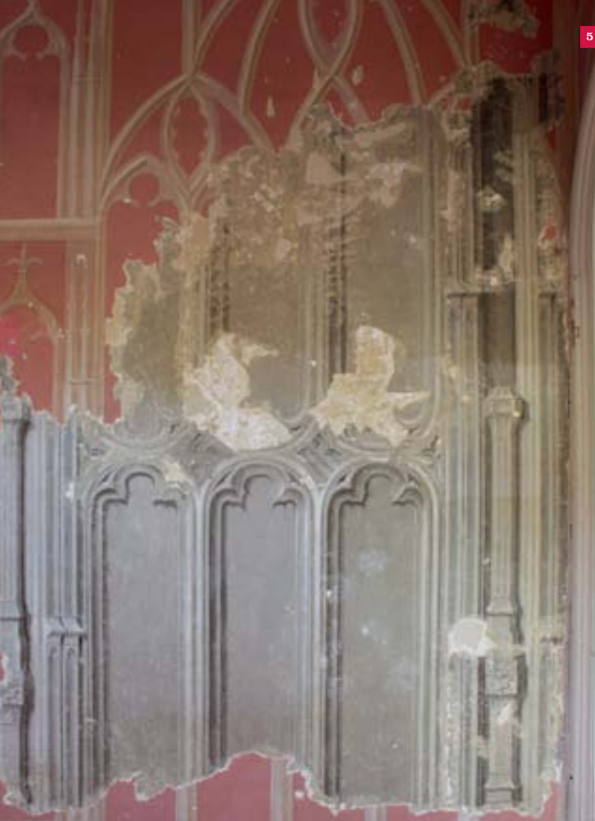
5 Walpole's original trompe l'oeil wall painting on the staircase revealed beneath modern decorations.
