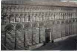
Pistoia • San Giovanni Forcivitas: facade conservation
