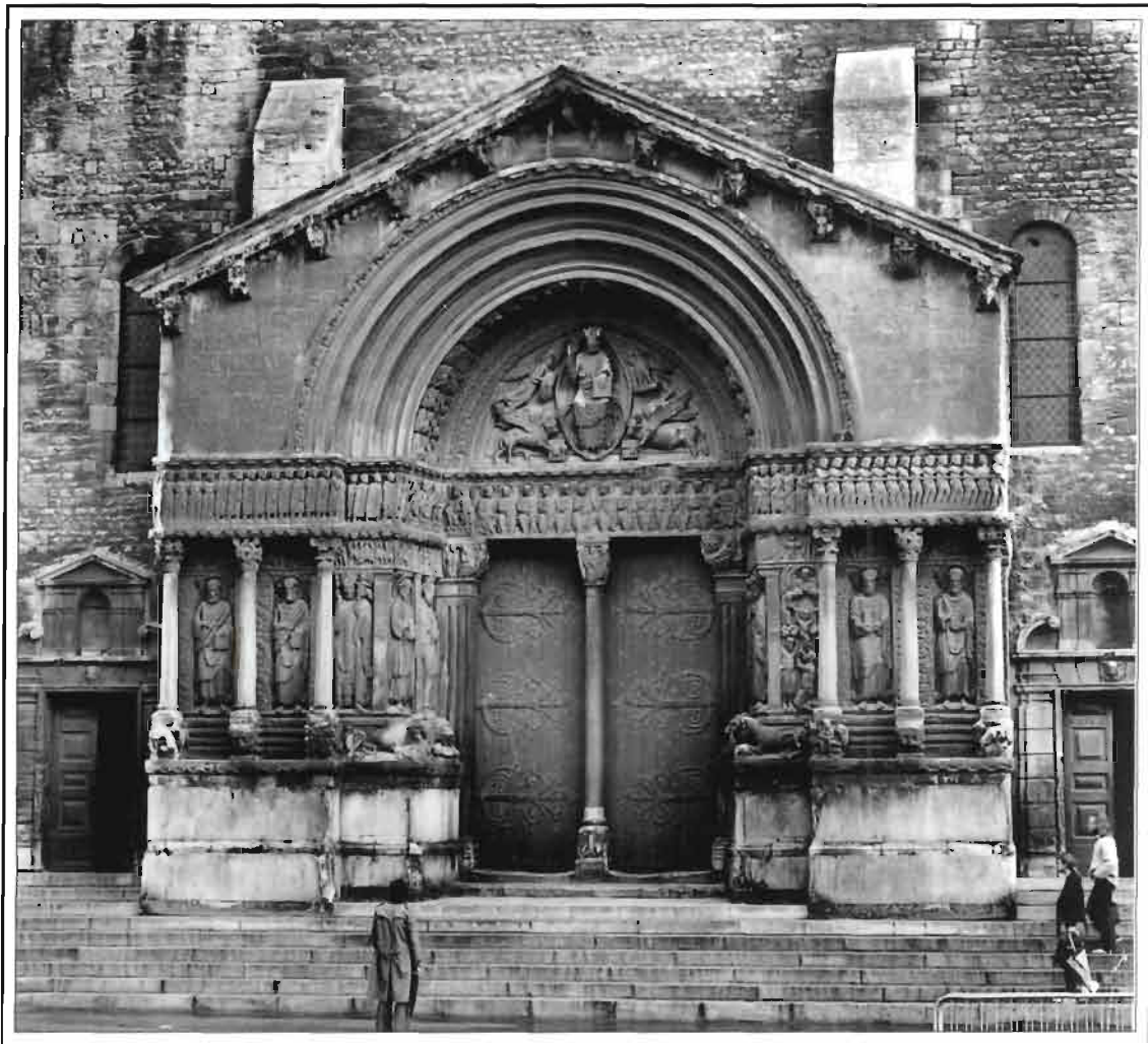
TOP: DETAIL OF THE TYMPANUM DURING RESTORATION BOTTOM: THE PORTAL BEFORE TREATMENT OPPOSITE: RESTORED FACADE AND PORTAL.
