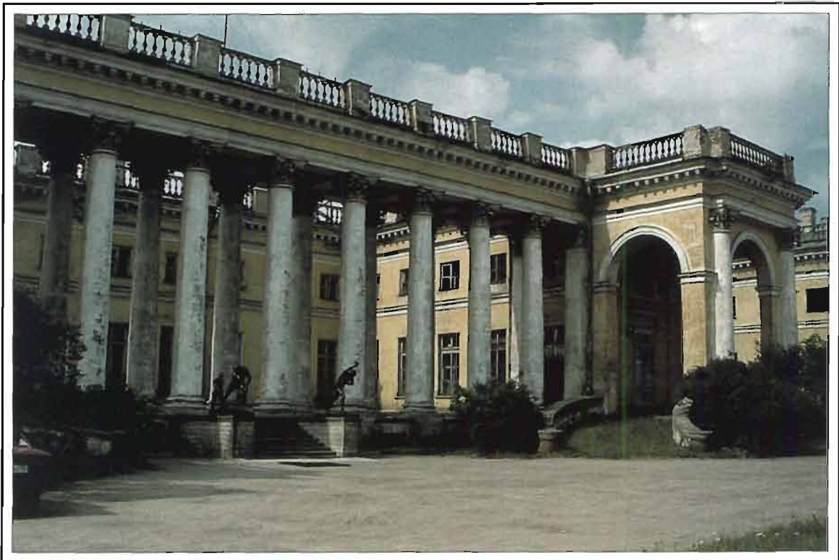
TOP LEFT: ALBERT MEMORIAL, LONDON TOP RIGHT: ST. GEORGE'S HALL, LIVERPOOL. VIEW OF GREAT HALL. ABOVE: ALEXANDER PALACE, ST. PETERSBURG, RUSSIA. DETAIL OF THE DOUBLE COLONNADE AT THE PRINCIPAL ELEVATION OF THE PALACE
