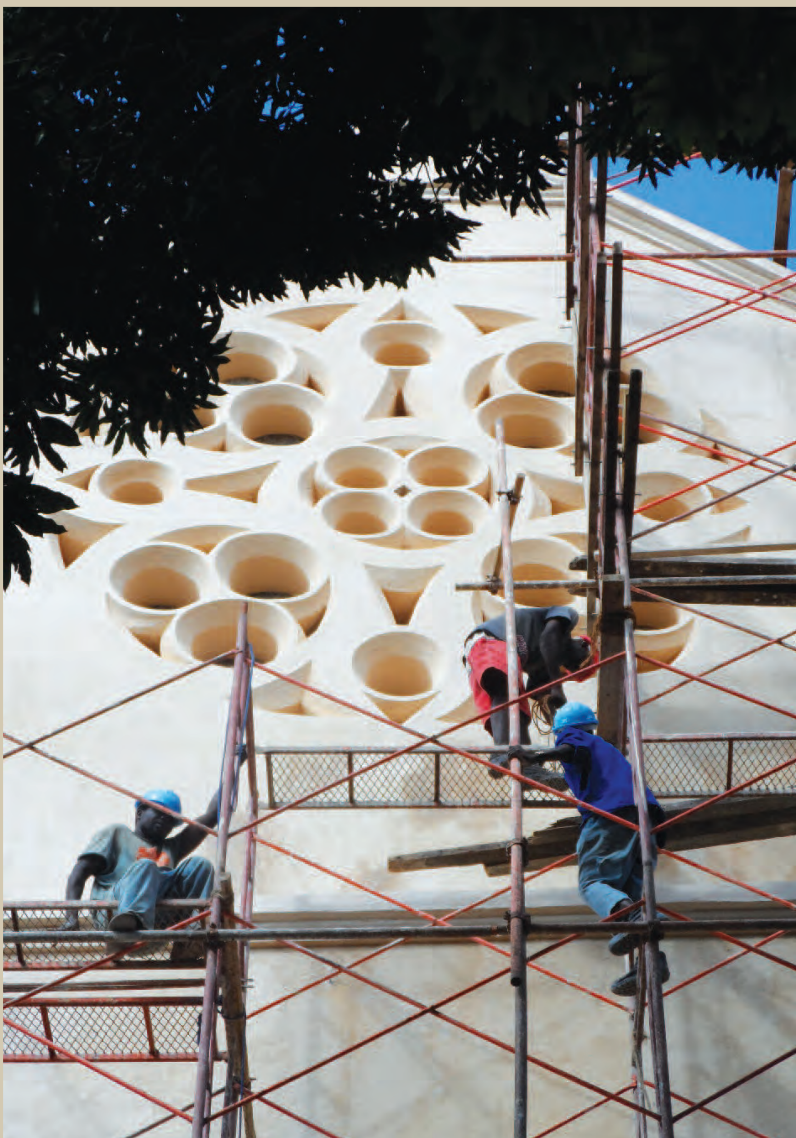
After: the restored rose window on the west gable wall.
