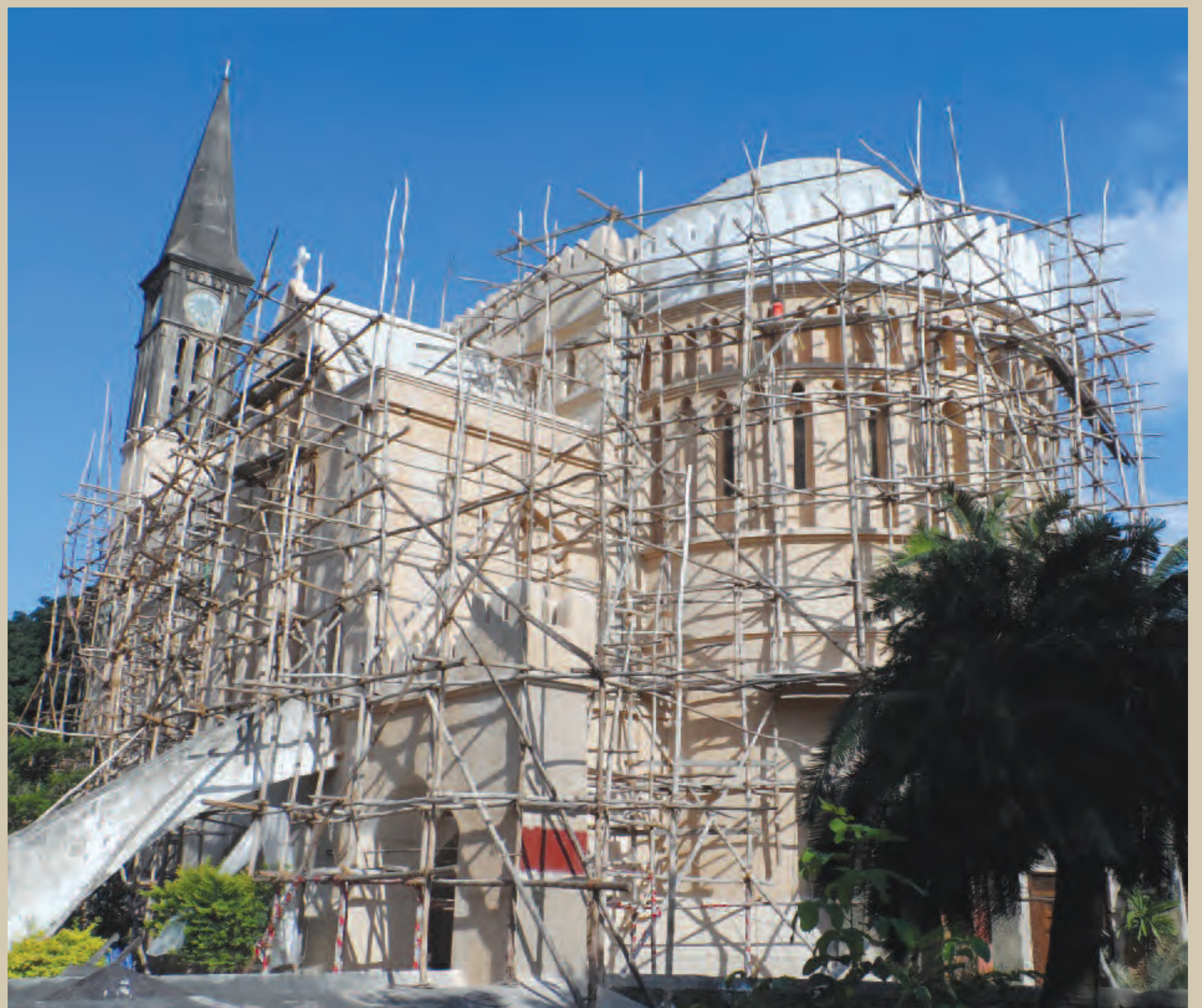
The cathedral in 2015 with conservation work underway.
