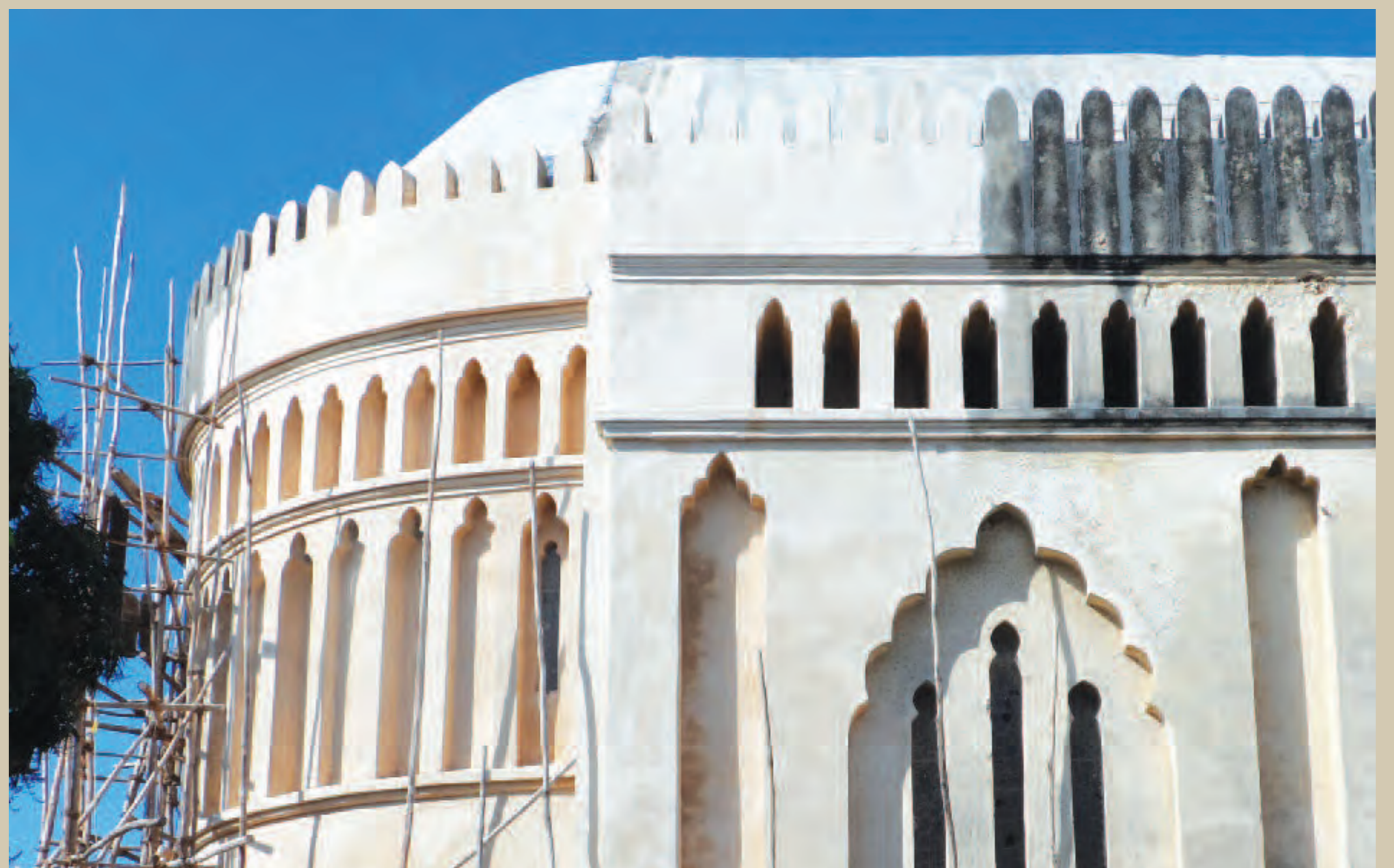
The east end, partially cleaned and with scaffolding in place. The pointed crenellations (top) are common on Arab houses, and the cusped arches (centre), reminiscent of mihrabs (semi-circular wall niches in mosques).
