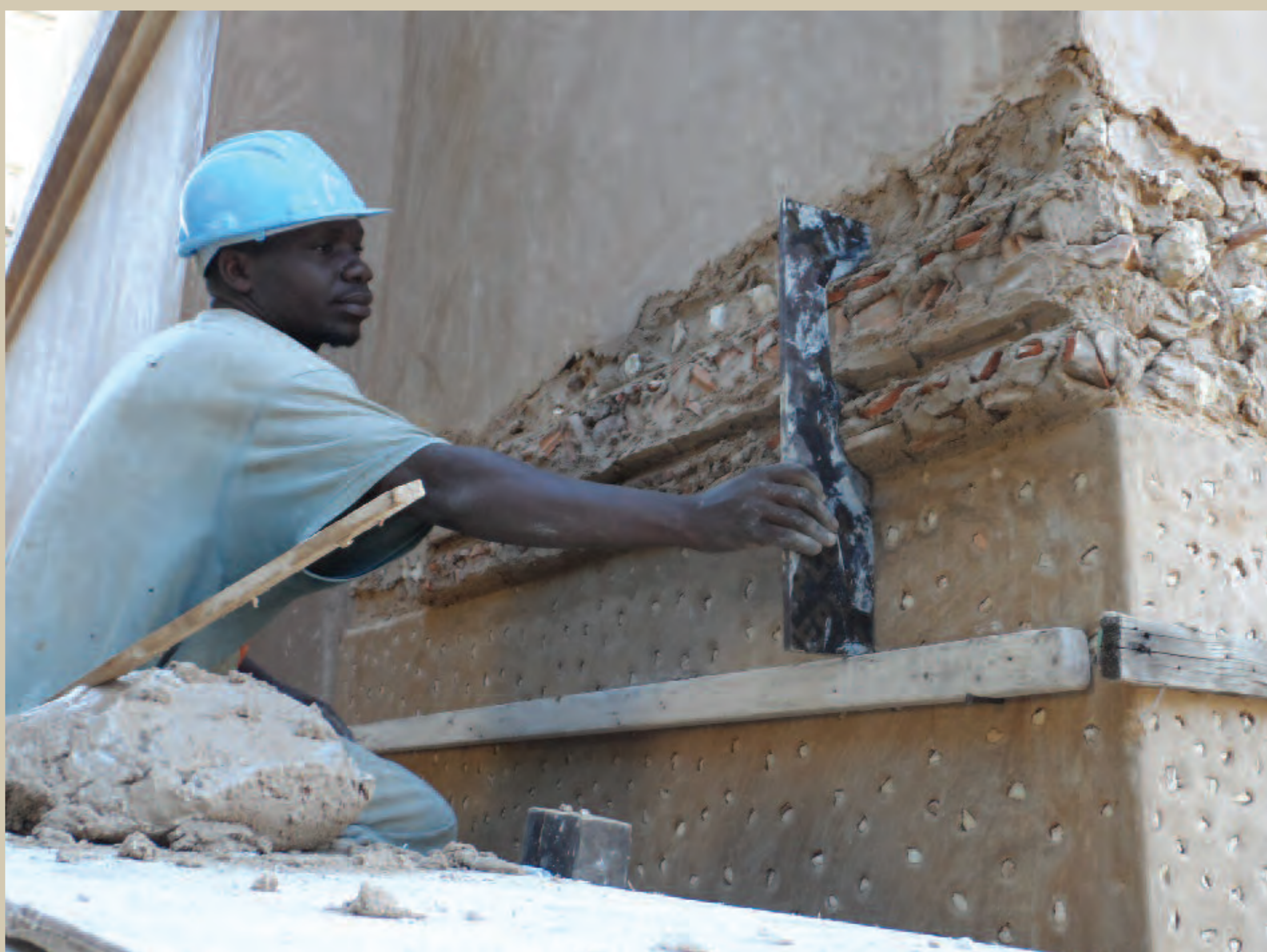
A craftsman recreates historic moulding profiles using a template.
