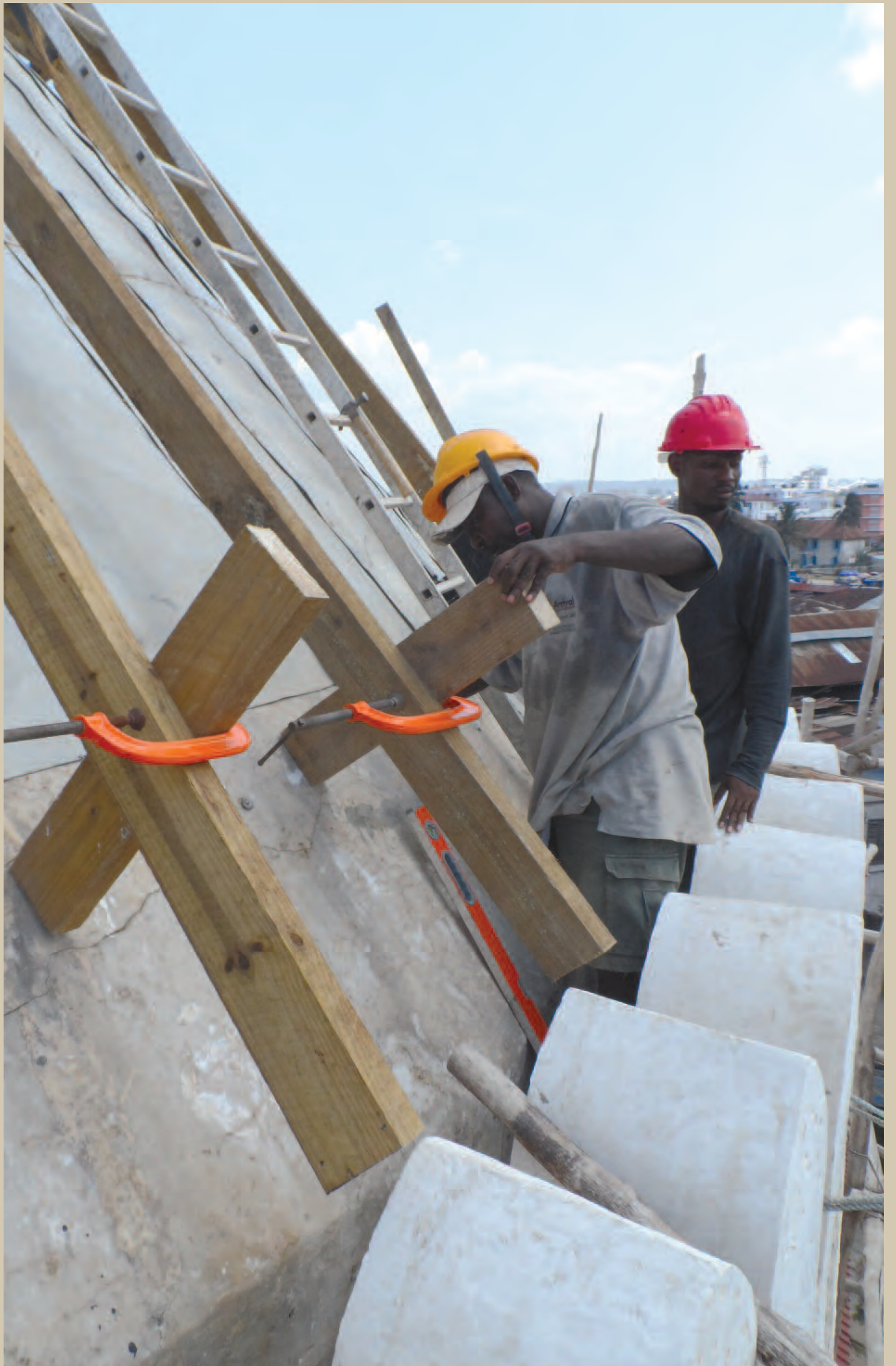
Conservation training in joinery techniques to construct the new roof.
