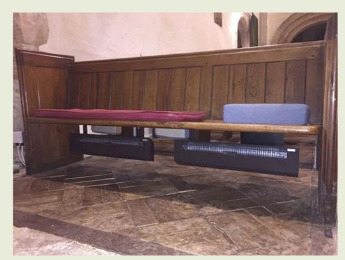
The oil boiler could have been replaced and extensive re-piping of the system would have been required to fix the underground leaks. This would have left the church on oil; the highest carbon fuel, releasing more greenhouse gasses per unit of heat than gas or electric heating. The heating project cost a total of £38k, with VAT being reclaimed through the Listed Places of Worship Scheme.
