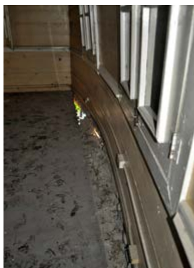
The timber frame of the second floor had shifted significantly on its masonry base during the earthquake;
