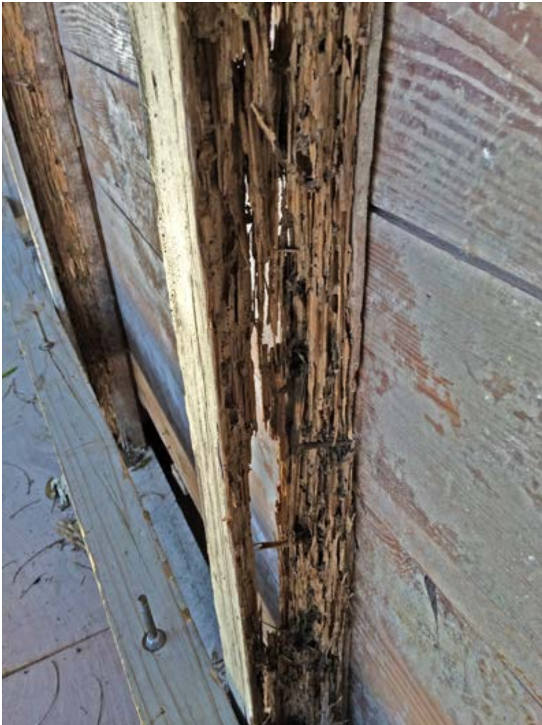
A wooden post on the eastern facade of the second floor had suffered heavy termite attack
