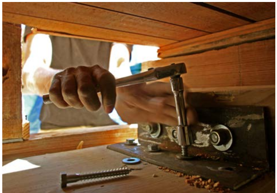
Installation of a plaque joining a tie rod to a sill on top of the masonry.
