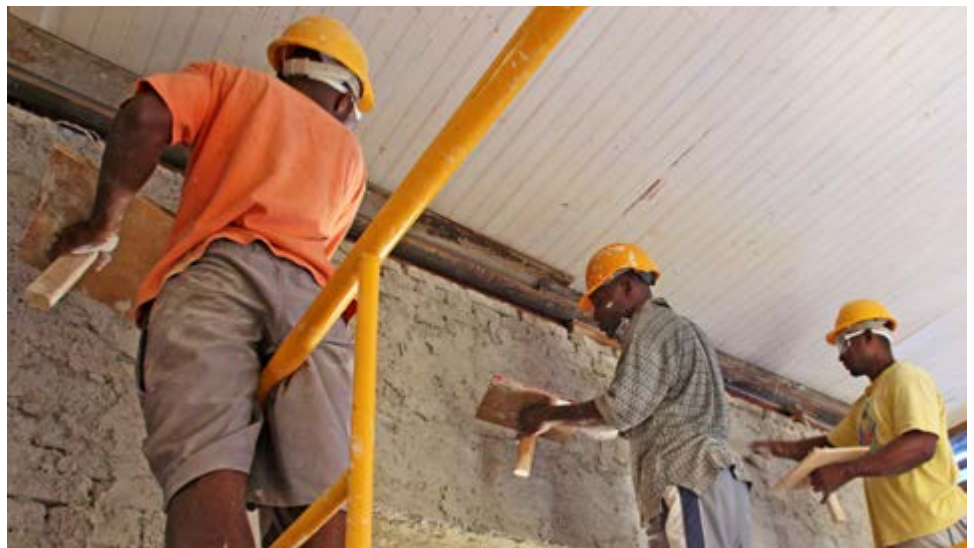
Eddy Pierret explains the process of preparing lime plaster to Marc Daniel, Jean Jacques and Donel Belenger; Jean Soner Delicat, Kenold Dutreuil, and Donel Belenger apply a scratch coat of lime plaster.
