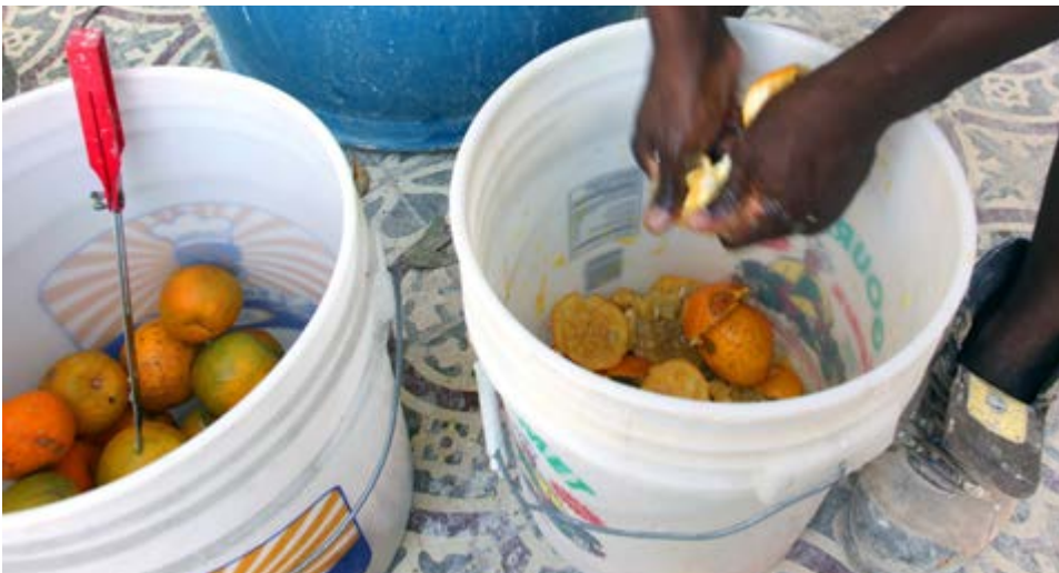
Patrick Lacroix demonstrates the appropriate mortar consistency for repointing; According to a Haitian technique, juice was extracted from sour oranges to provide an additional binder for the lime wash; Bijou Lifite applies a coat of lime wash.
