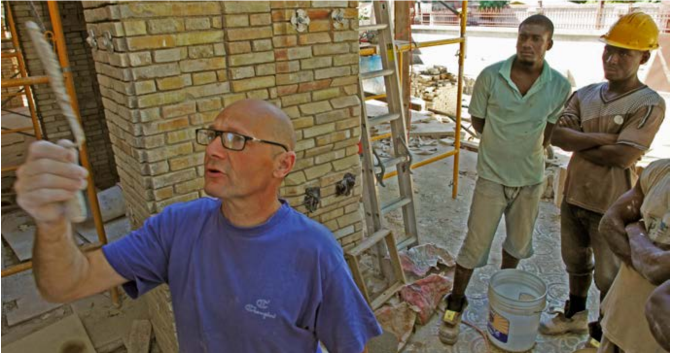
Patrick Lacroix demonstrates the appropriate mortar consistency for repointing; According to a Haitian technique, juice was extracted from sour oranges to provide an additional binder for the lime wash; Bijou Lifite applies a coat of lime wash.
