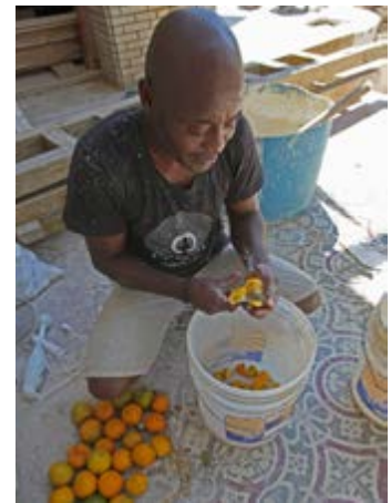
Kénold juices bitter oranges to prepare a Haitian formula for whitewash.
