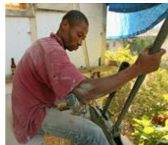
Bruno uses a Tirfor come-along winch to realign the house on its foundation.
