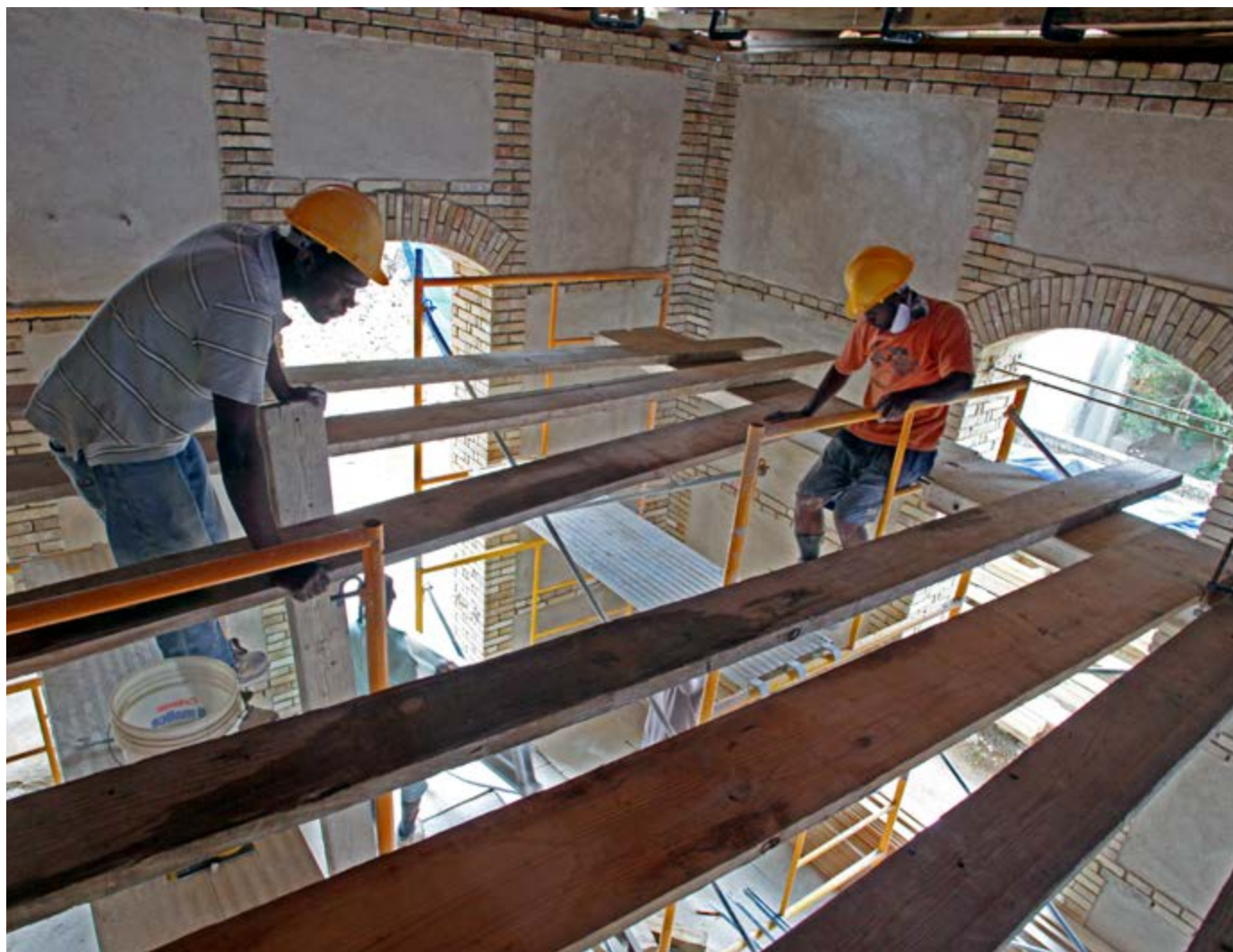
Above: The team assembles scaffolding prior to installing the seismic reinforcement.
