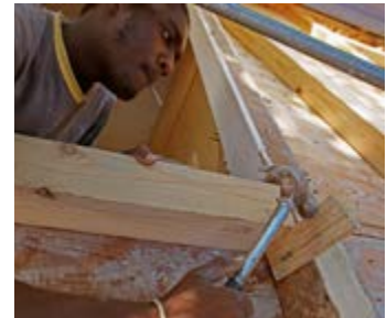
Bijou uses a shim to accurately align floor beams.
