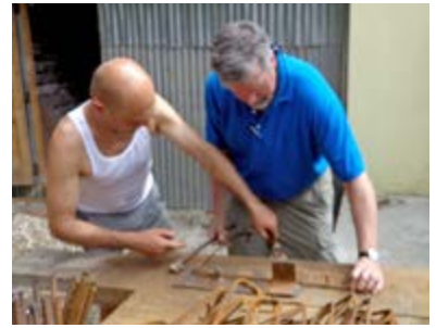
Patrick Lacroix from IPW and Steve Kelley from WMF work together to prepare rebar reinforcement for the foundation of the house.
