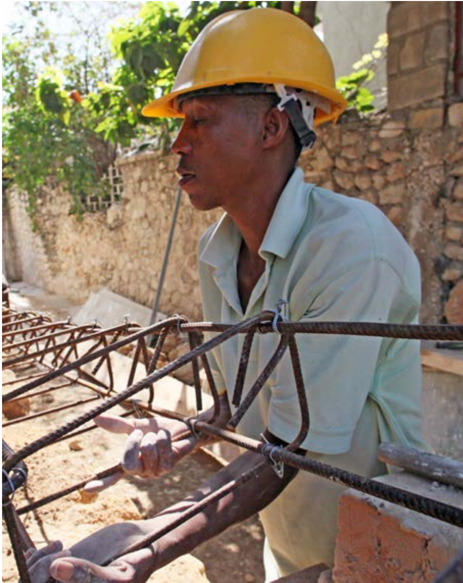
Casimir installs the rebar for the foundation of the west gallery.
