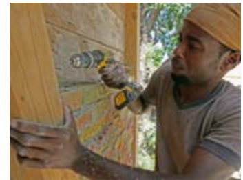
Lefevre inserts small rods to reinforce the second-floor masonry.
