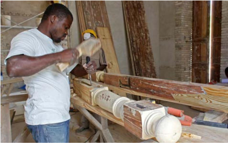
Jean Louis Augustin works to repair a post from the original staircase; Jean Louis Augustin, Pety and Ricardeau repair a section of the banister; on the second floor, a small balcony was installed around the stairwell.
