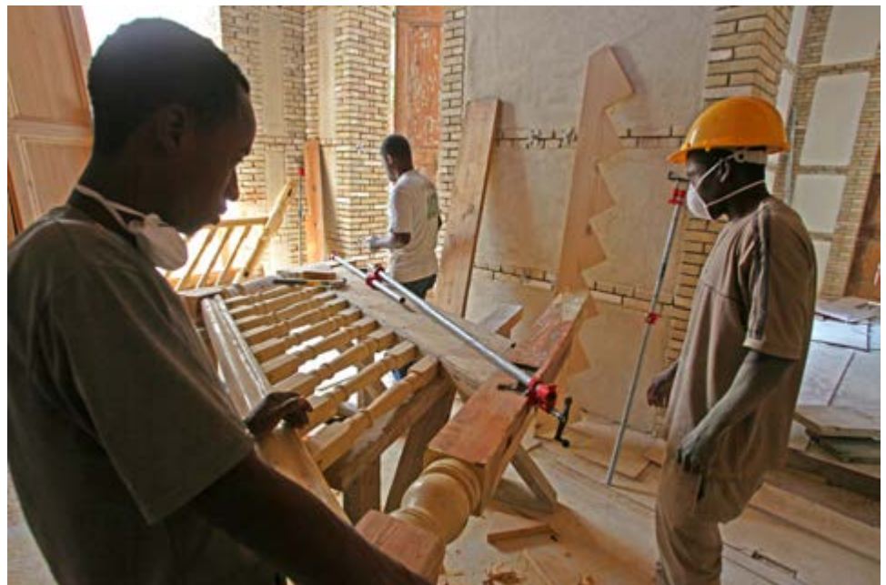
Jean Louis Augustin works to repair a post from the original staircase; Jean Louis Augustin, Pety and Ricardeau repair a section of the banister; on the second floor, a small balcony was installed around the stairwell.
