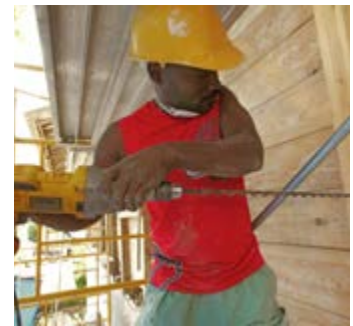
Héril reinforces the house's timber frame with steel rods.
