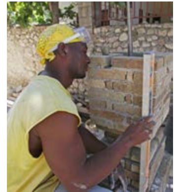
Bélanger checks that a pillar in the west gallery is plumb.
