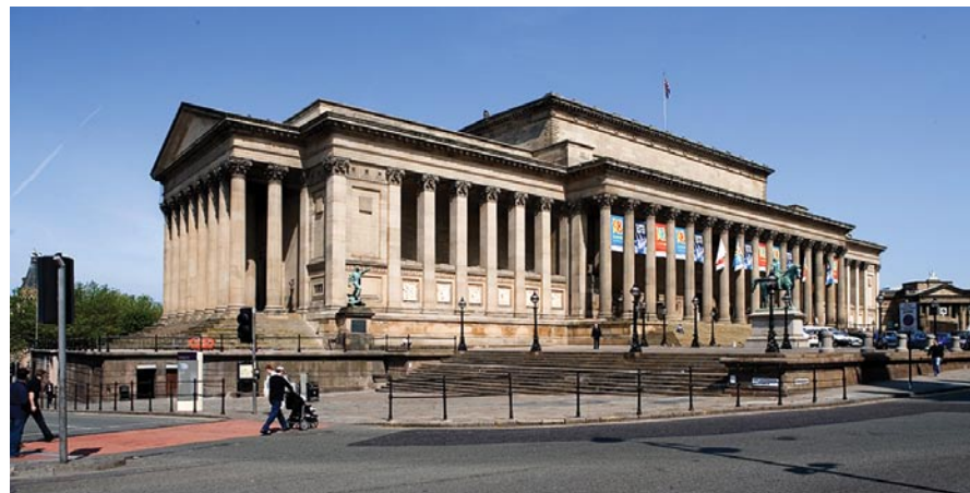
THE CLASSICAL GRANDEUR OF ST. GEORGE’S HALL, BELOW, OUTSIDE AND IN, HAS MADE IT A LIVERPOOL LANDMARK. LEFT, A PAINTER RESTORES THE HALL’S CEILING PANELS TO THEIR ORIGINAL COLORS.
