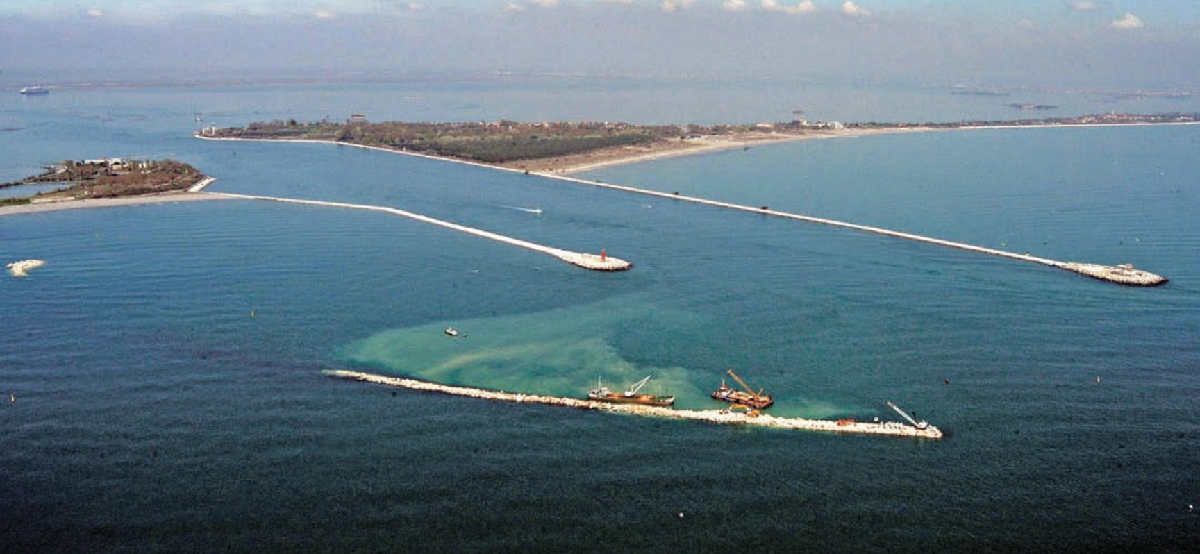
At the Malamocco inlet, above, one of three through which the Adriatic enters the lagoon, construction of a breakwater in preparation for the installation of the MOSE barrier system (see page 28) began in 2003. A scale model of the lagoon, left, is used to assess the impact of the barrier system.
