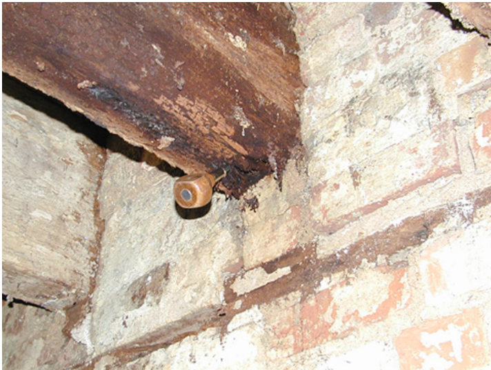
Figure 11. Probing with an awl at the interface between a timber beam and an exterior wall
