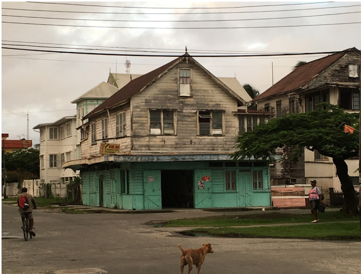
Figure 8. Weathered wood in need of paint; the wood surface must be properly prepared before applying additional paint or the new paint will fail via flaking and peeling
