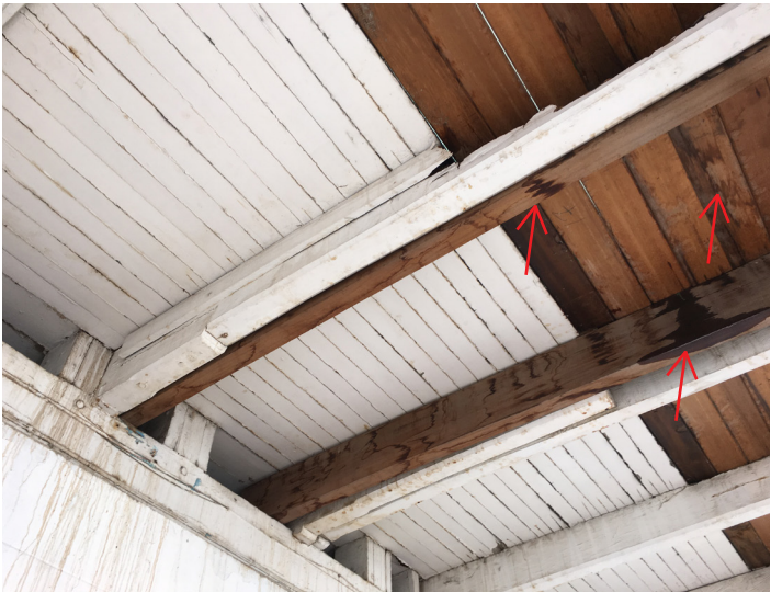
Figure 10. Moisture stain on the rafters and porch roof sheathing due to leaks in the porch roof (Courtesy of National Trust of Guyana)
