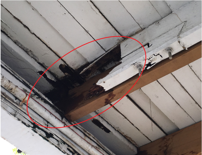
Figure 9. Decayed wood due to poor moisture drainage from the porch roof (Courtesy of National Trust of Guyana)
